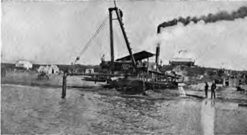
CAPE NOME HYDRAULIC MINING CO.'S BEACH MACHINE AT WORK.
